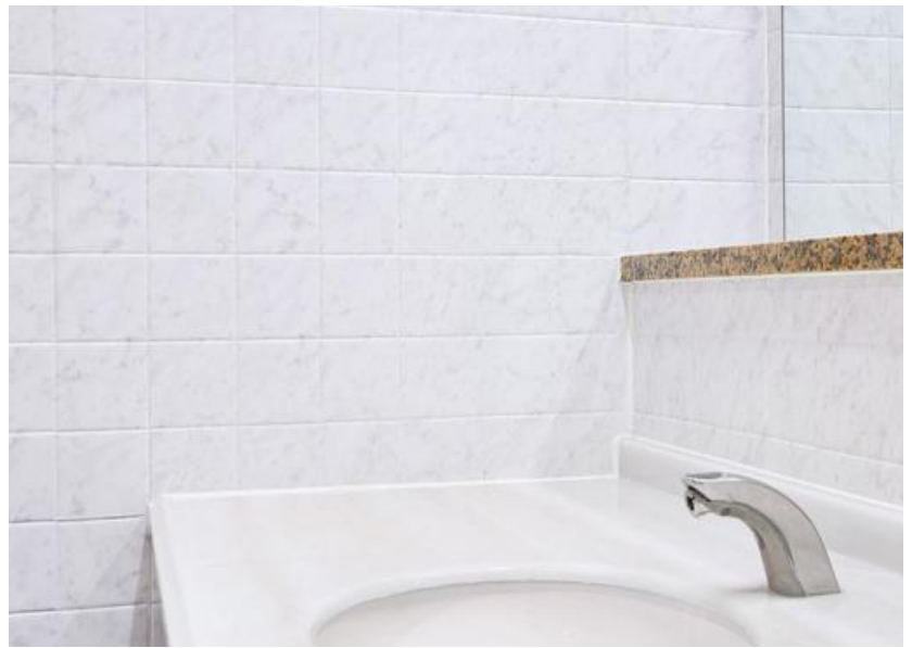
Restroom refurbishment / ST-024TIL
